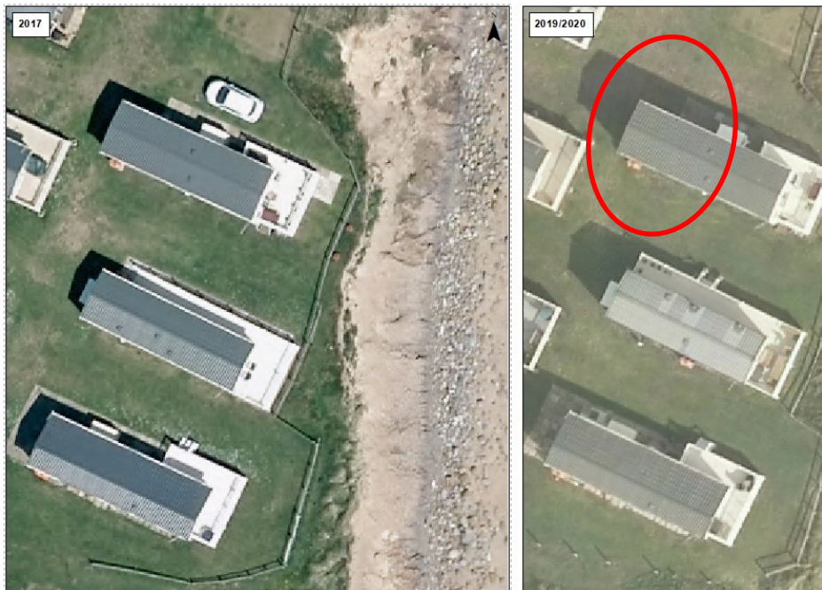
Figure 2-13 – Cliff erosion at Sandy Bay Caravan park, 2017 (left) and 2019-20 (right)
