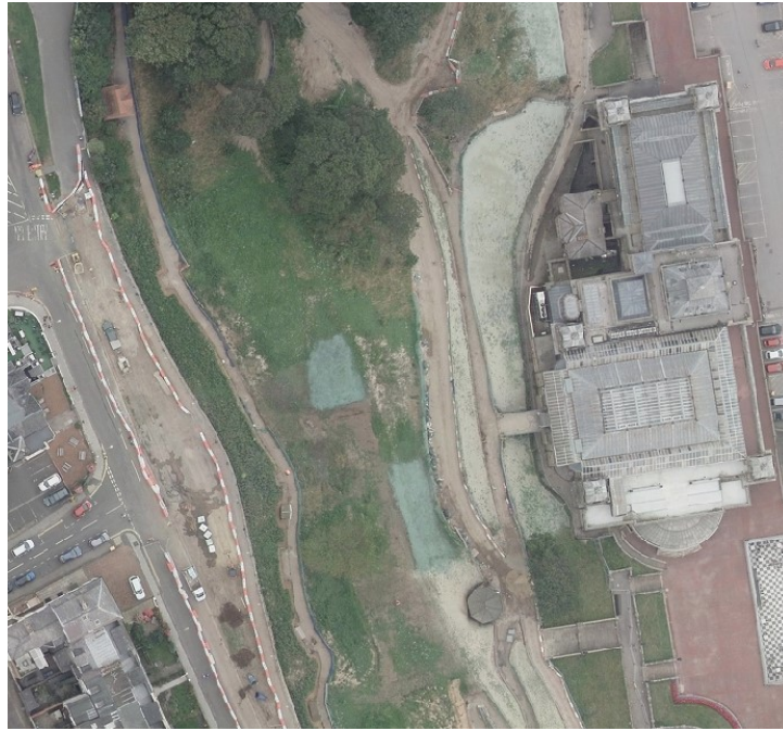
Figure 2-24 – Stabilisation works to cliffs behind Scarborough Spa during 2019-20 survey
