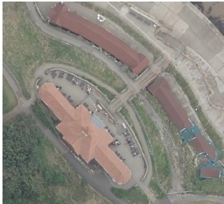
Figure 2-24 – Damaged beach huts by Clock Tower Café captured during the 2019-20 survey
