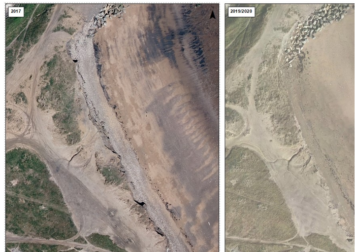
Figure 2-10 – Erosion of colliery spoil cliffs south of Lynemouth Power Station revetment, 2017 (left) and 2019-20 (right)
