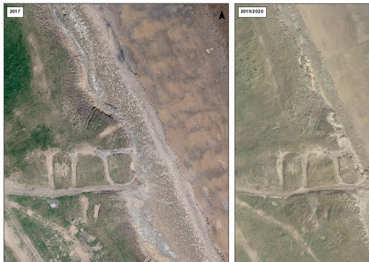
Figure 2-9 – Erosion of colliery spoil cliffs in Lynemouth Bay, 2017 (left) and 2019-20 (right)
