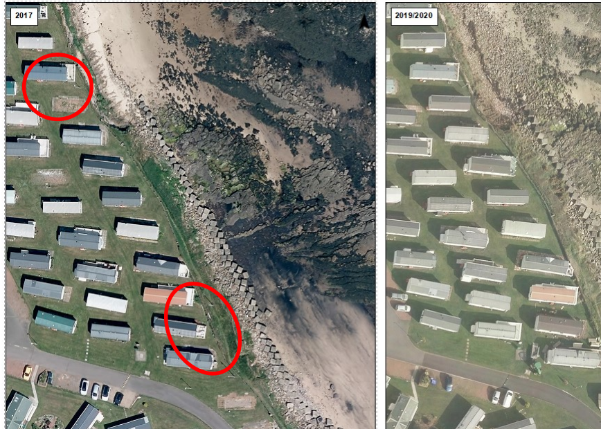
Figure 2-11 – Caravans previously removed from eroding cliff edge before 2017 now replaced, 2017 (left) and 2019-20 (right)
